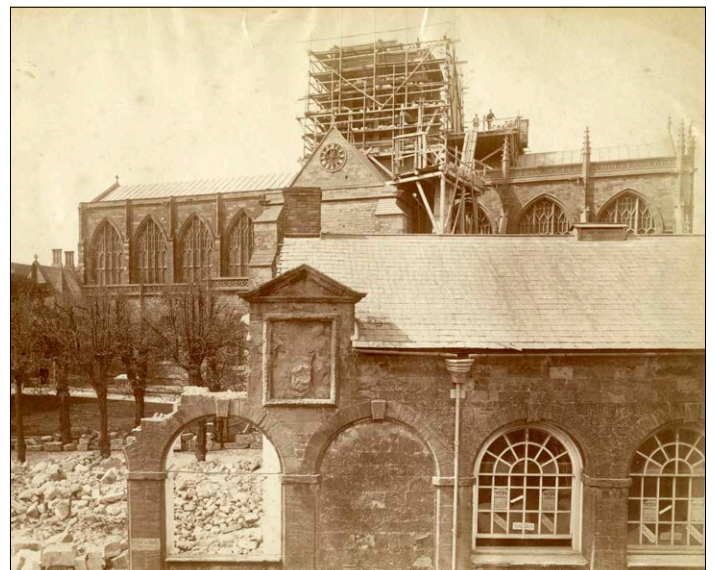
The 1883 renovations showing the partly demolished Town Hall in the foreground
